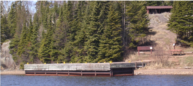
Chippewa Harbor Dock
